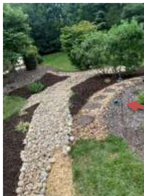
Erosion control added at 478/476
