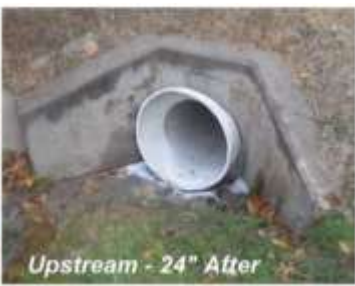
An example of what we will expect to see after the resin pipe is in place
