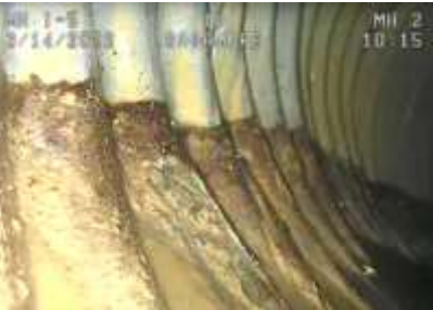
Typical corrosion of our storm water pipes
